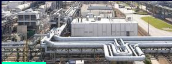
Electrification, Automation & Digitalization solutions
