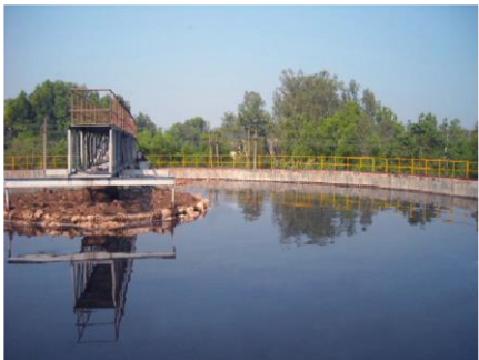
Primary Clarifier - Paper
