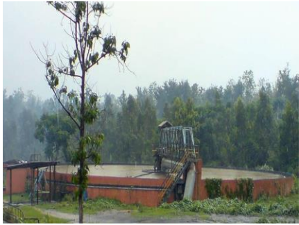
Primary Clarifier - Pulp
