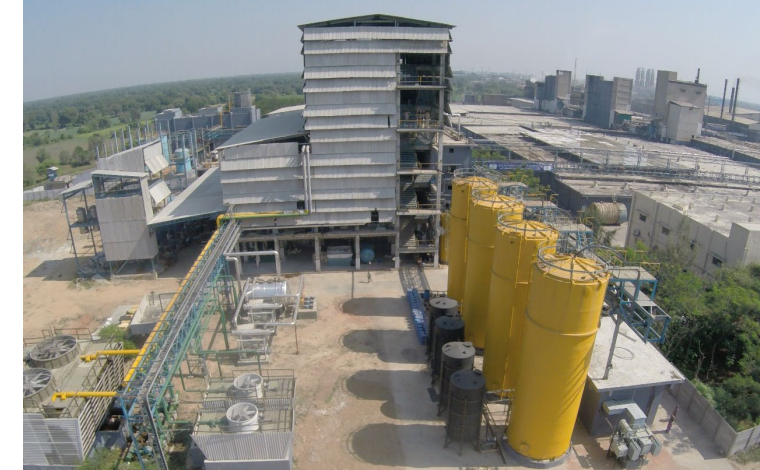
Multiple Effect Evaporator Plant (MEEP)
