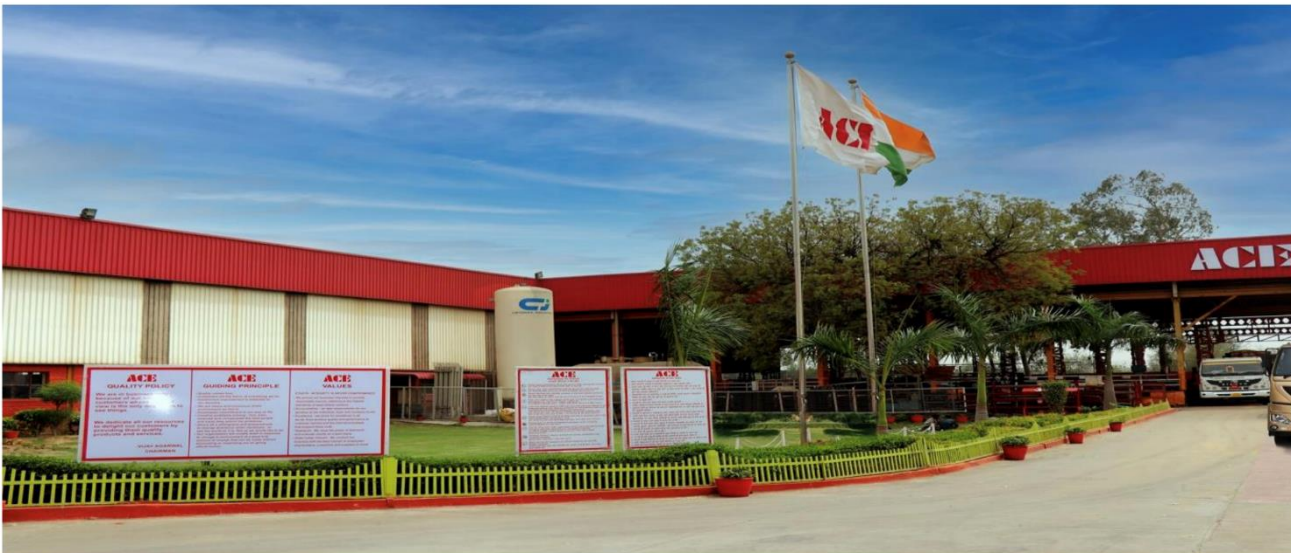
Fabrication Unit and Weld Shop
