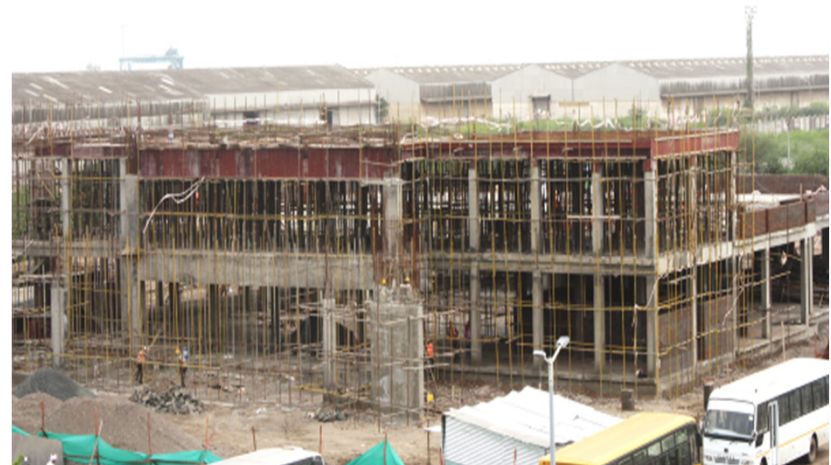
Construction of Office Building Commenced
