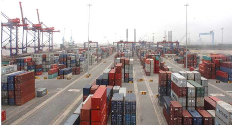
Container Yard Works- Complete & in use
