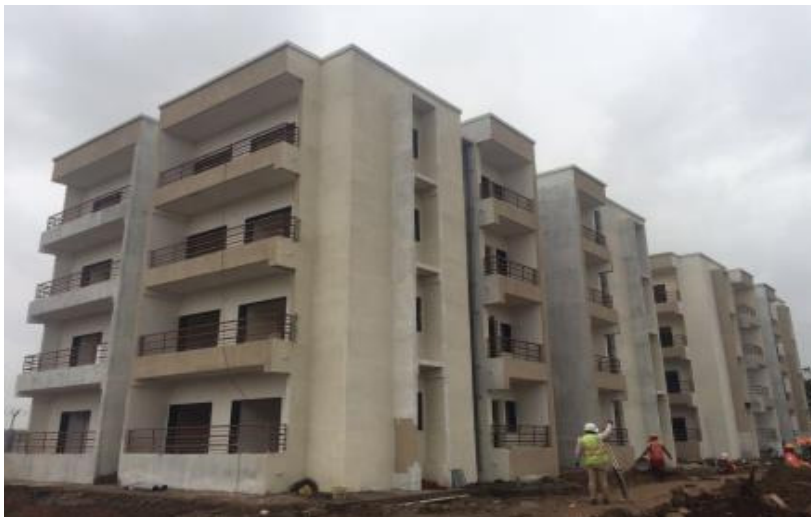
Construction of Residential Building
