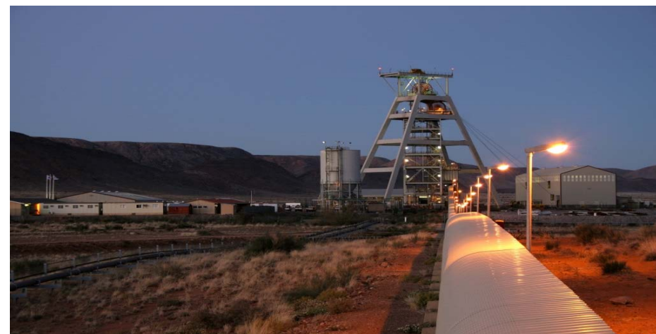
Deeps Shaft at Black Mountain Mining, Aggeneys
