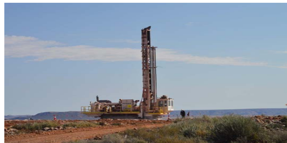
Blast haul drilling at the greater Gamsberg area
