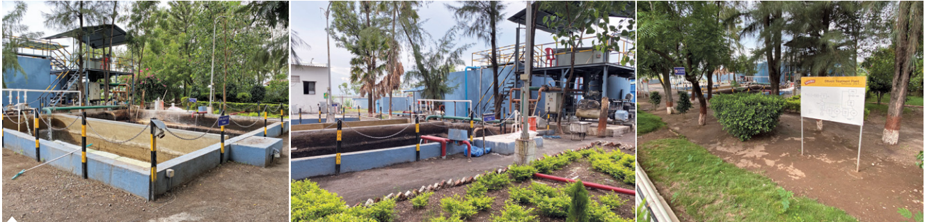
Effluent Treatment Plant
