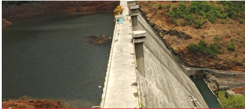
Ghatghar Dam – Maharashtra 84m high 10th fastest completed dam in the world an India's first RCC Dam
