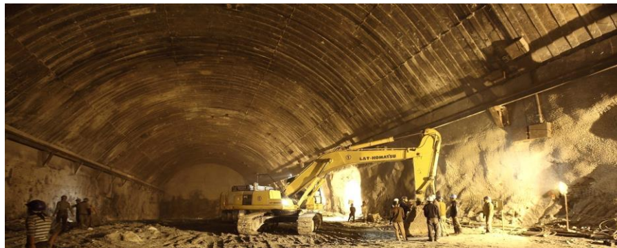
Srisaillam HE Project - Andhra Pradesh (900MW) Largest Underground Cavern in Asia 25.7m (W) x 53m (H) x 236m (L)
