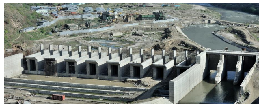
Sawrakuddu HE Project - Himachal Pradesh (111 MW) First Piano Key Weir in India
