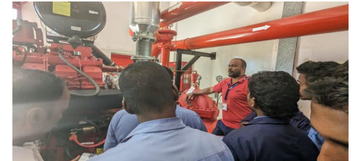
Fire Hydrant Pump training at Hosur Plant by OEM
