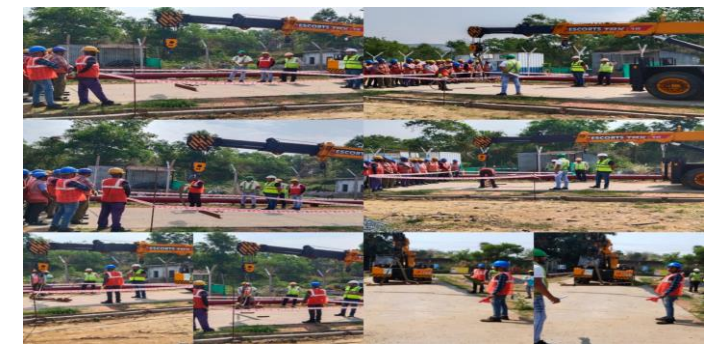
Onsite Safe Lifting Operation training at MPL Dhanbad site
