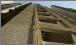
Galvanised Iron Installation
