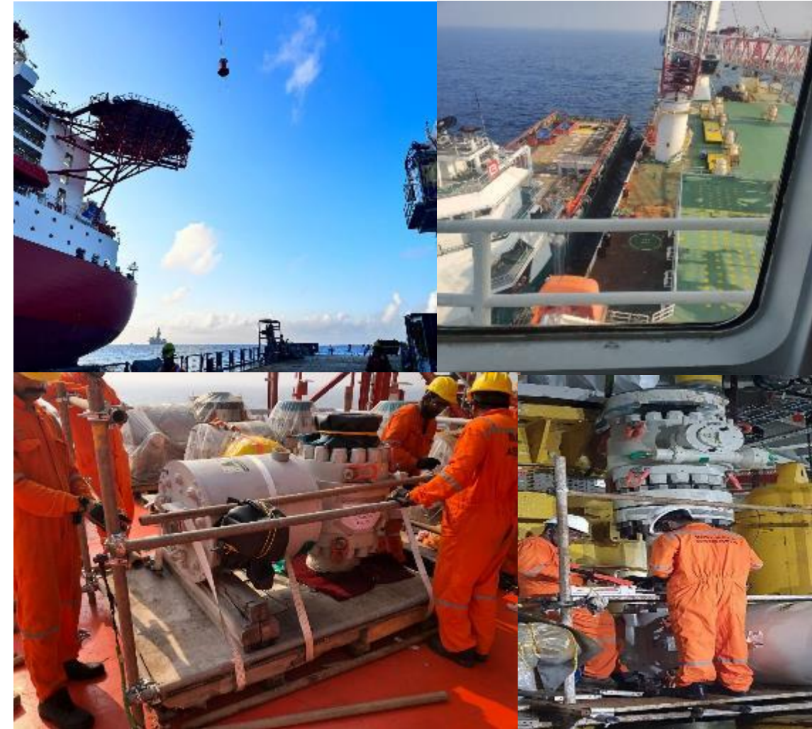
MJ FPSO Hookup & Field Installation Pictures
