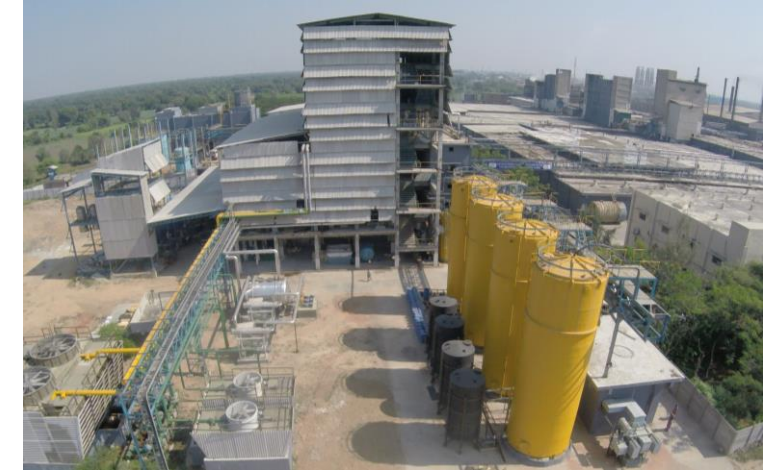
Multiple Effect Evaporator Plant (MEEP)
