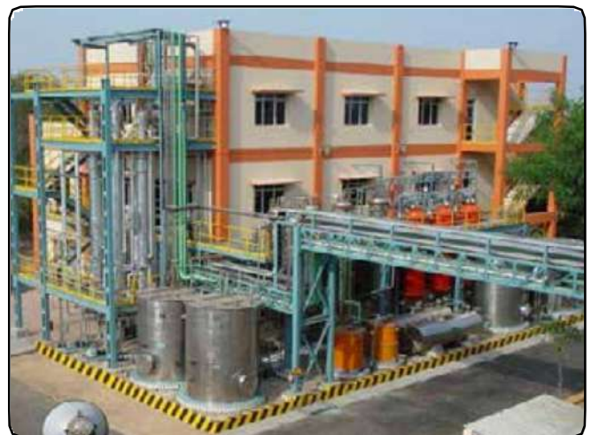
A section of the Fine Chemicals Plant
