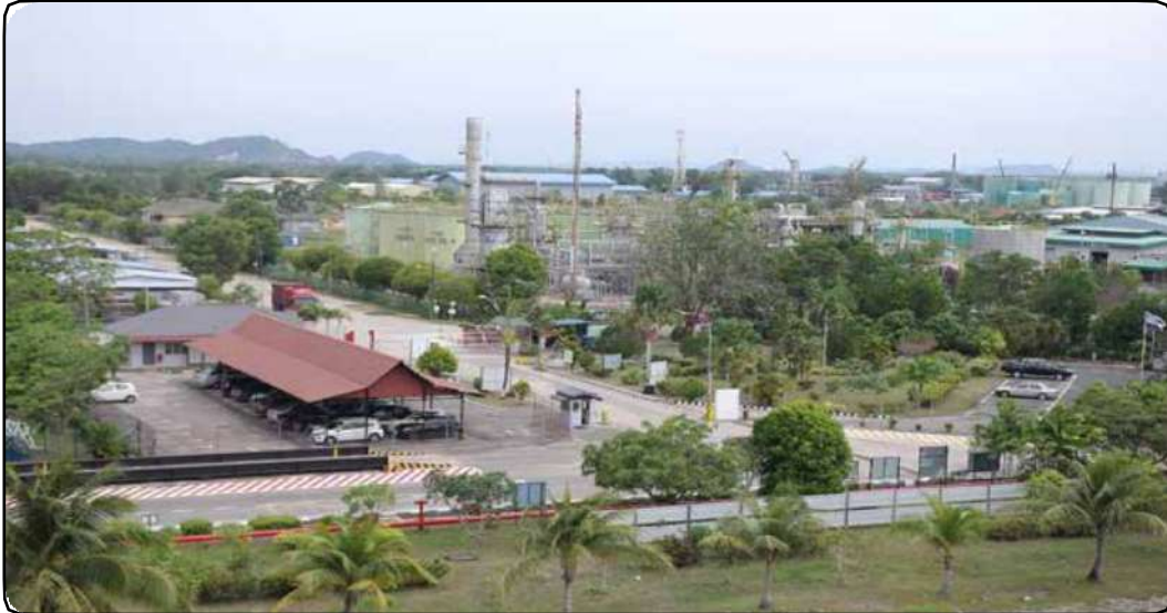
Overview of our subsidiary in Malaysia - The Maleic anhydride Plant
