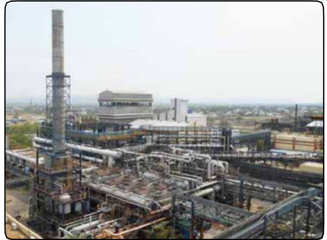
PA Plant - Ranipet, during revamp
