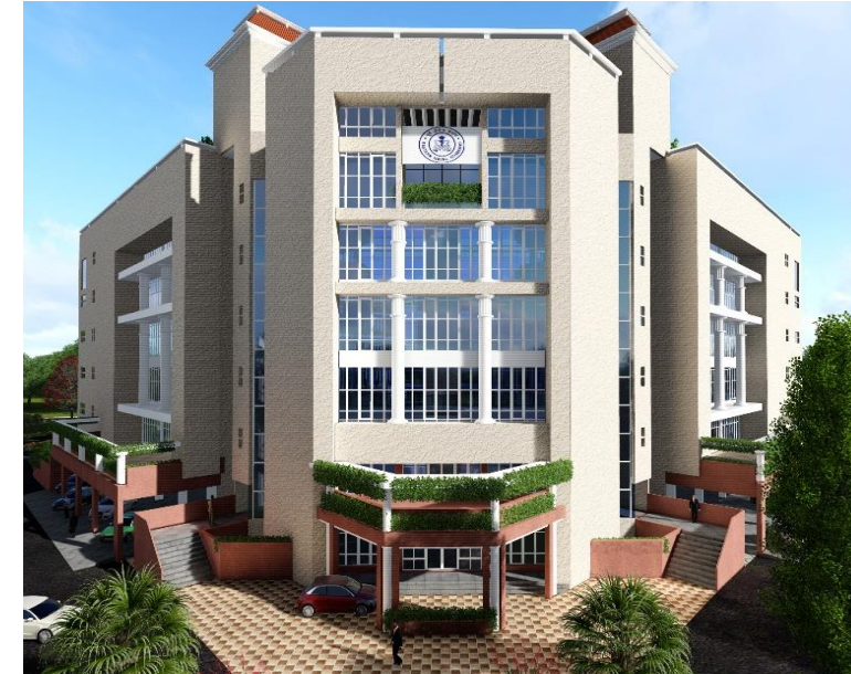
Civil works for a Defence client
