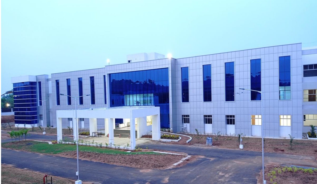
Data centre project, Defence client
