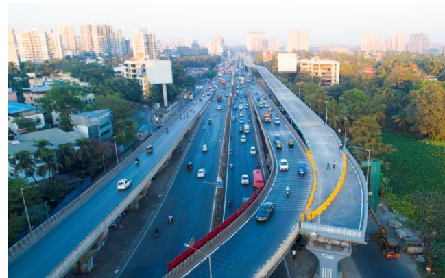
Chheda Nagar Flyover Part 1
