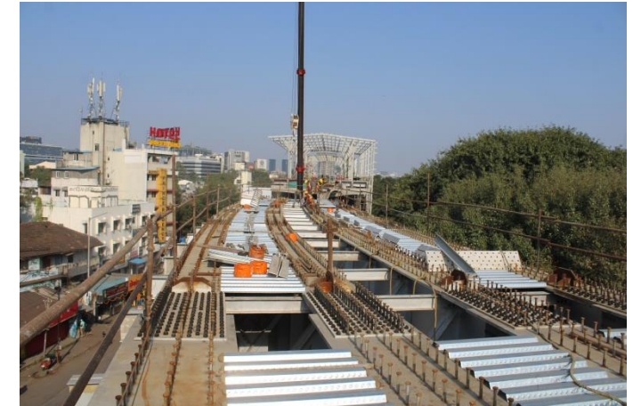
Pune Elevated Metro
