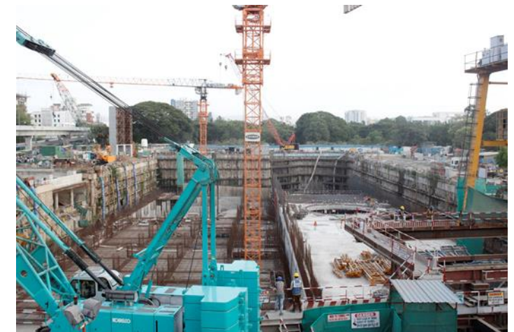
Pune Underground Metro
