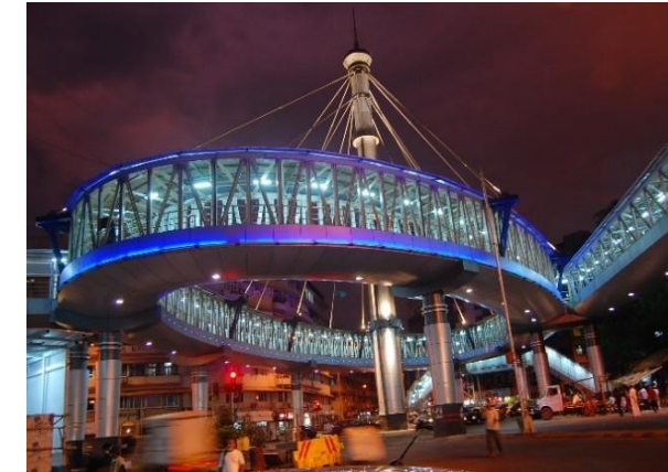
Grant road Skywalk
