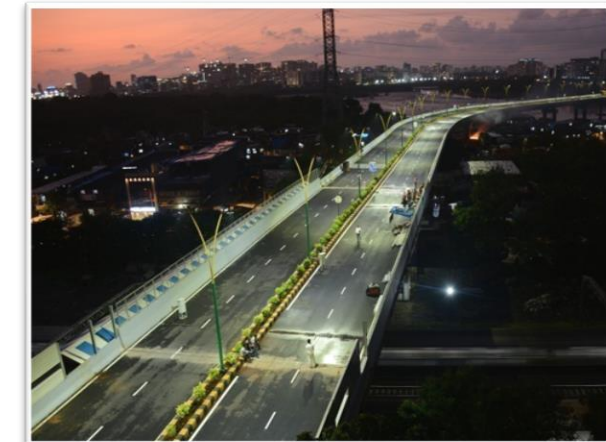
BKC- Chunabhathi Flyover
