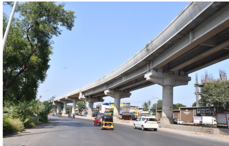
Mumbai Metro Line 6
