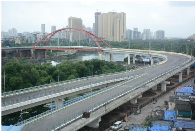
Kalwa Bridge Thane
