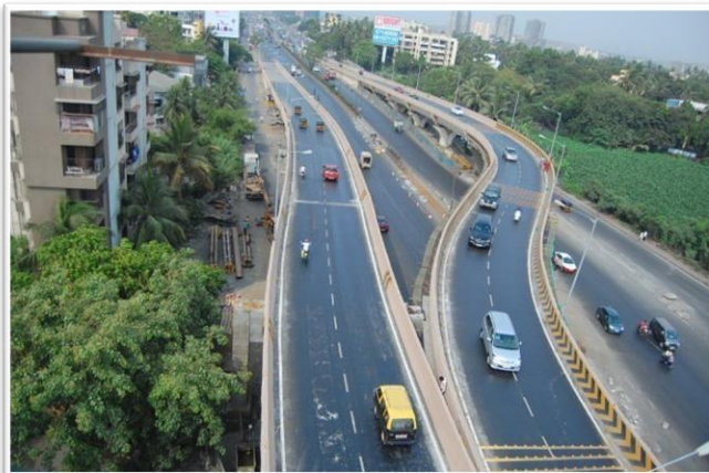
Amar Mahal Flyover
