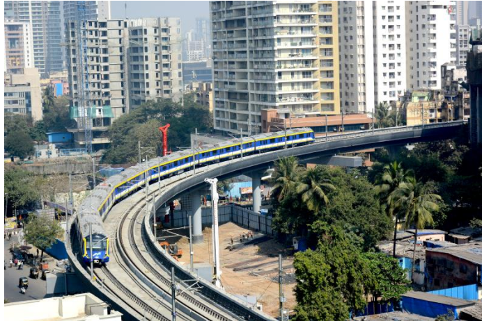
Mumbai Metro Line 2A
