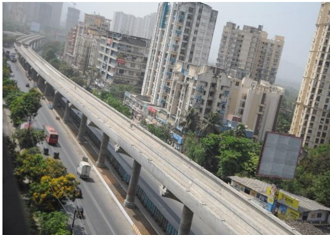
Mumbai Metro Line 4A
