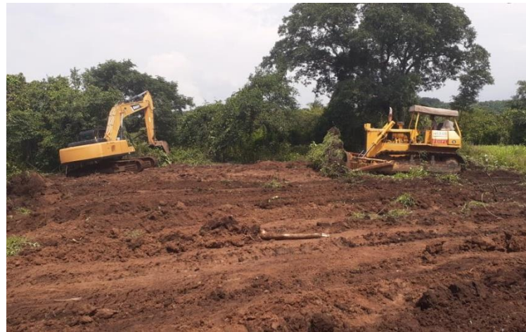
Vadodara Mumbai Expressway, IRCON
