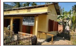
PUBLIC UTILITY AREA CONSTRUCTION
