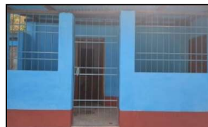
SCHOOL BUILDING RENOVATION
