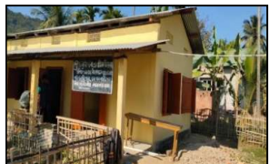
SCHOOL BUILDING RENOVATION
