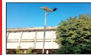
SOLAR STREET LIGHT
