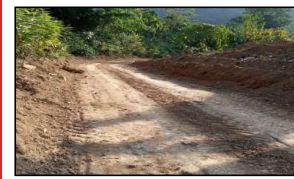
PUBLIC UTILITY AREA CONSTRUCTION
