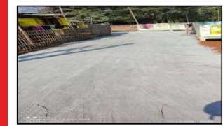
CONSTRUCTION OF RCC ROAD
