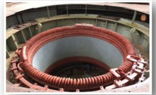
Implementation of Hydro Electric Project, 2 MW at Upper Kallar, KSEB
