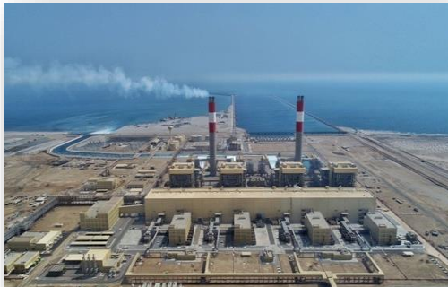
4X660 MW Shuqiaq SSPP, KSA (Completed Project)
