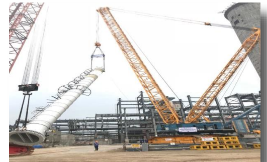
Urea Reactor Tank Installation At Ramagaundam, Telangana
