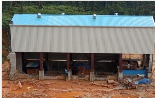
Implementation of Hydro Electric Project (2MW/5.14 Mu)-KSEB
