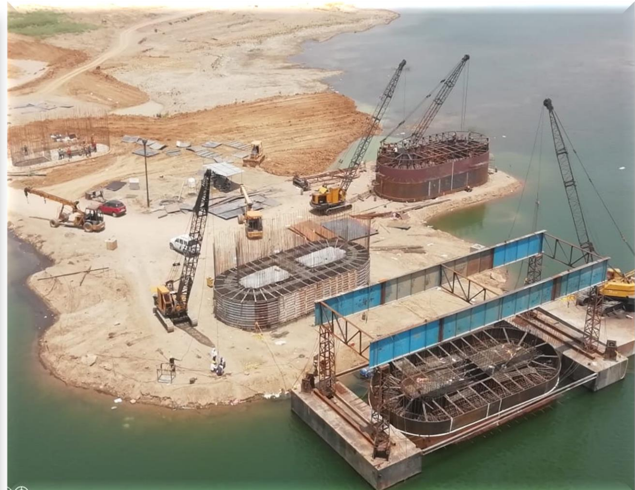
Dhaulpur Project Executed Caissons for Double - D well foundation in a perennial river Condition
