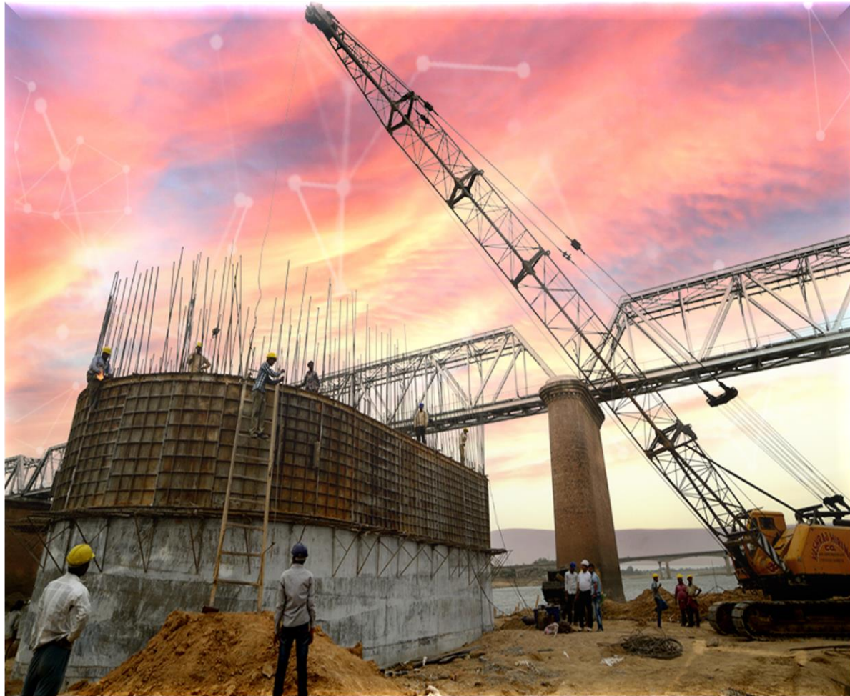
Kalpi Project Constructing railway bridge
