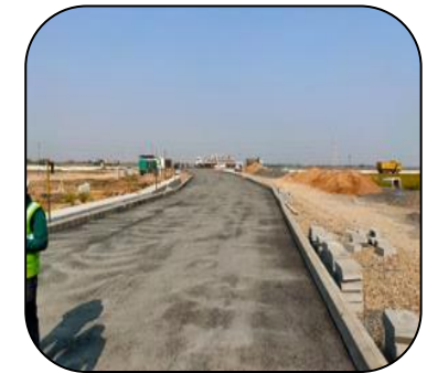
Under Construction Site
