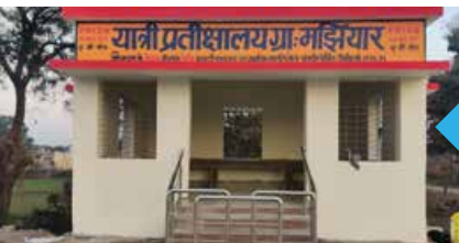
Construction of Bus Shelters at Majhiyar Village
