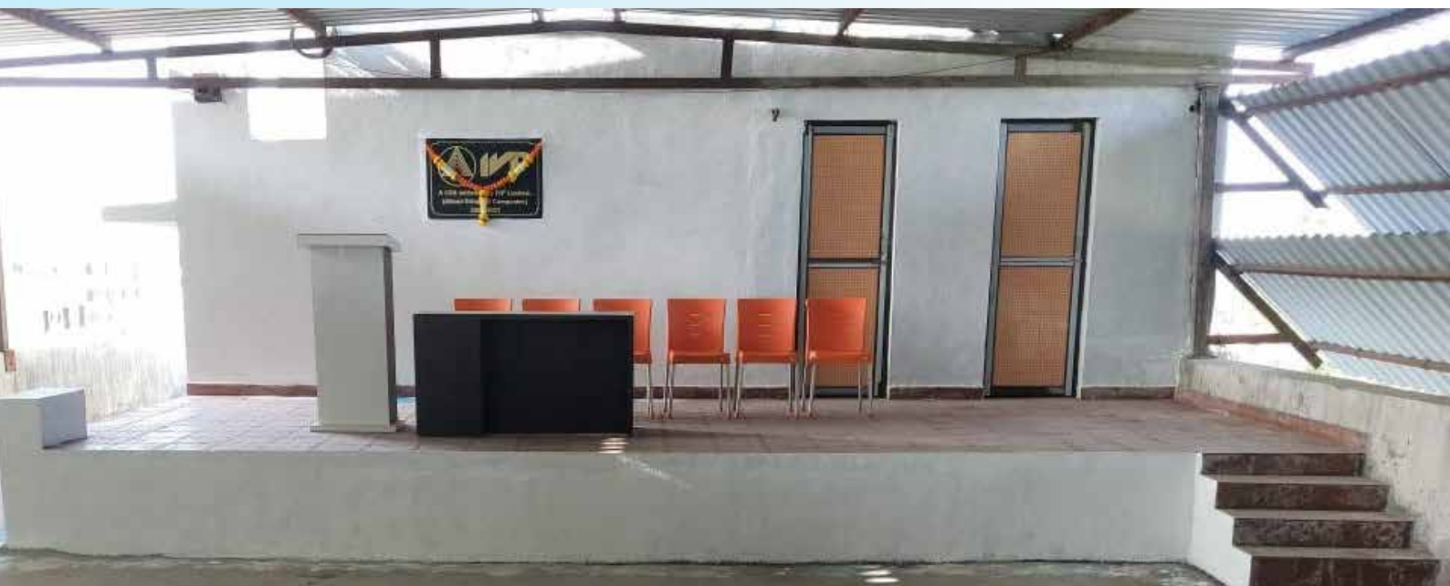
New Auditorium constructed in Seva Ashram School, Boisar, Palghar
