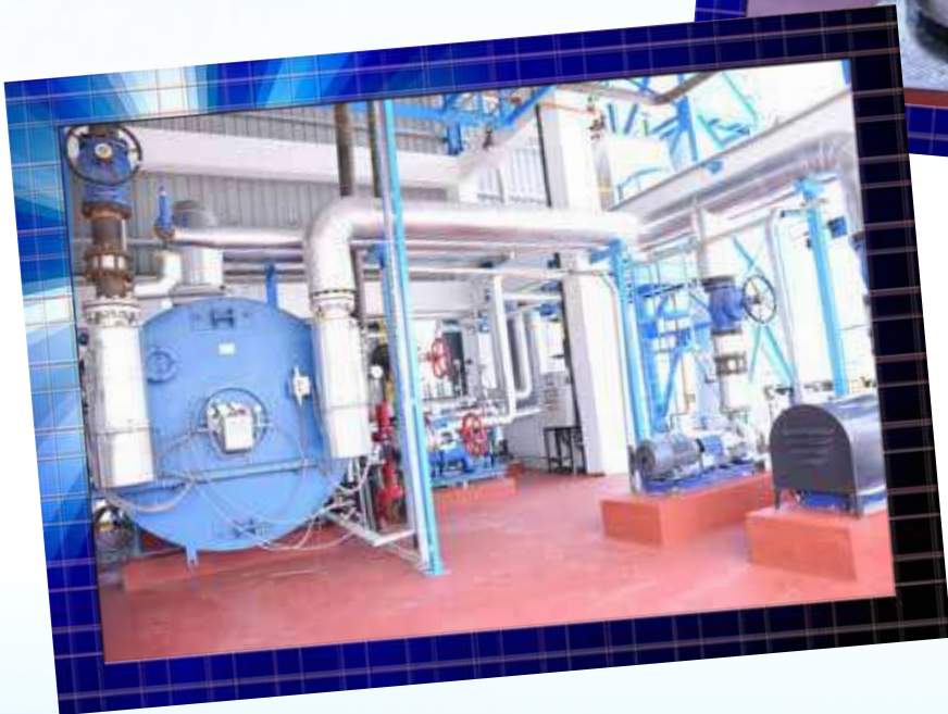
Tarapur Manufacturing Unit II
