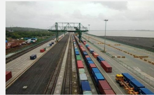
Bharat Mumbai Container Terminal (BMCT) – PHASE 1, Navi Mumbai
