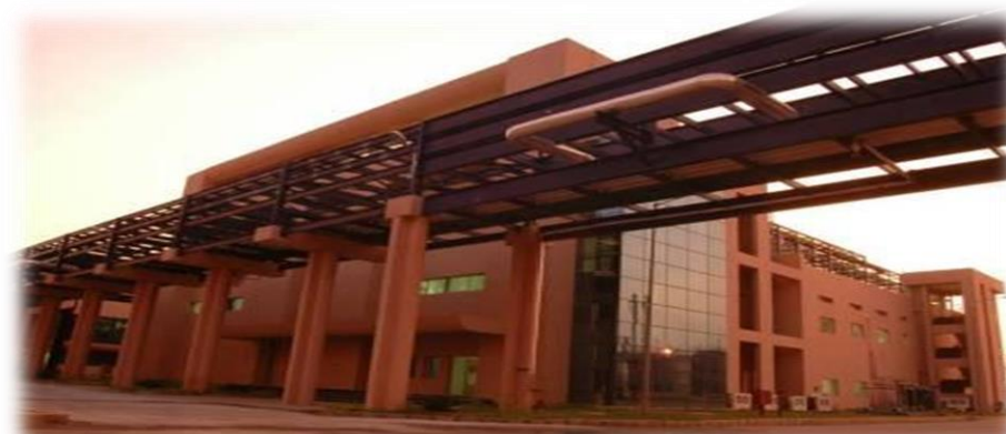
Syngene's USFDA approved manufacturing facility at Bengaluru
