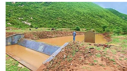
Water Conservation Project
