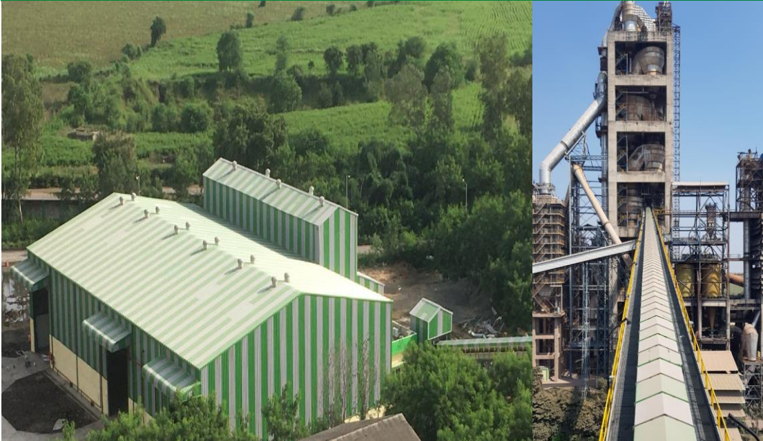
AFR Project commissioned in January 2022
