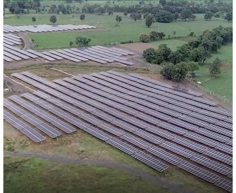
5.5 MW Solar Project ready
