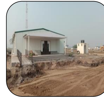
Under Construction Site
