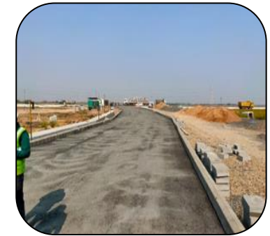
Under Construction Site
