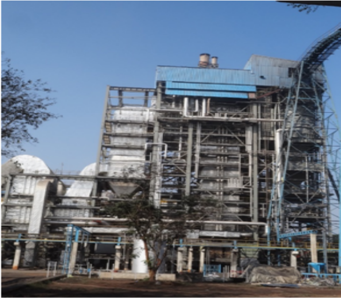
60 MW Captive Power Plant
