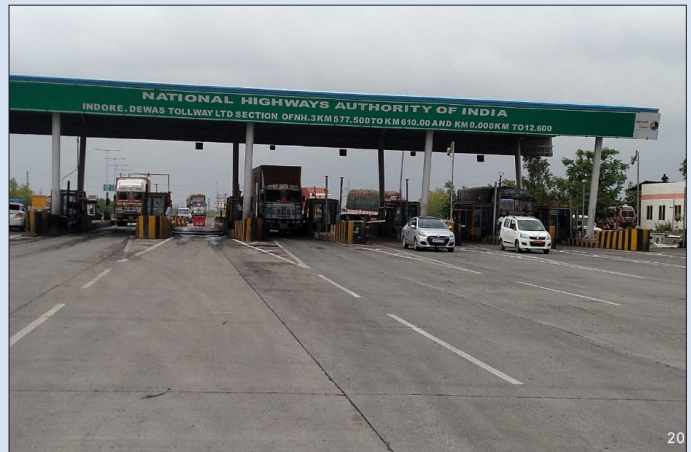
Indore Dewas Tollways Limited
