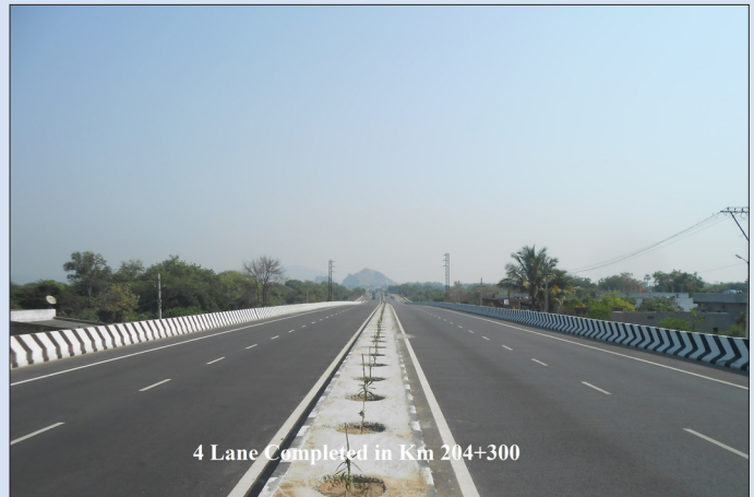
HKR Roadways Limited
