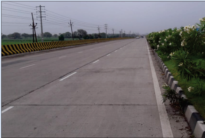
Indore Dewas Tollways Limited
