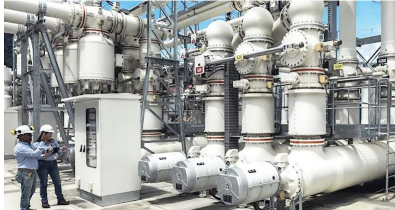
Power quality solutions commissioned across cement, mines, ports
