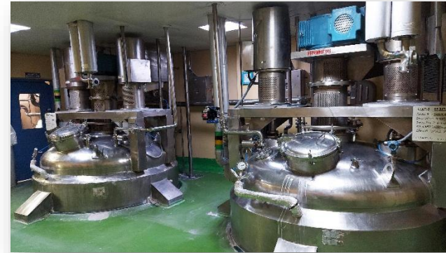
Main Mixing Tank
