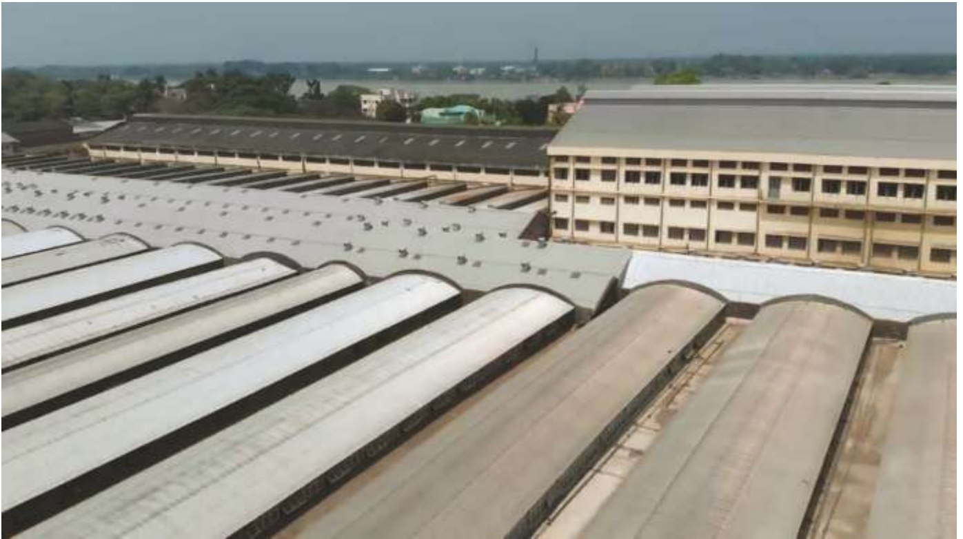
Jute mill located at Budge Budge
