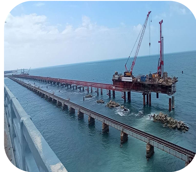
Pamban Rameswaram bridge in Tamil Nadu
