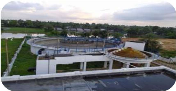
Water treatment project in Agartala, Tripura
