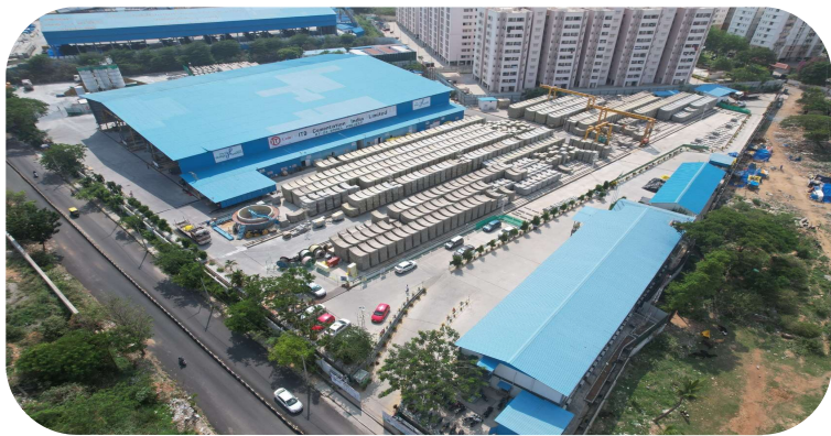
Bengaluru underground metro casting yard
