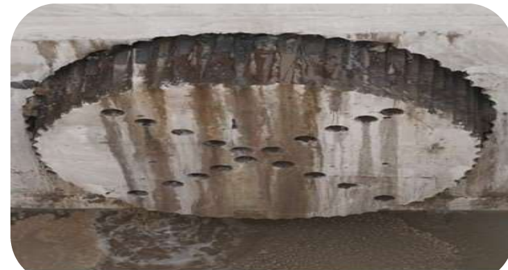
MCGM micro tunnel breakthrough in Mumbai
