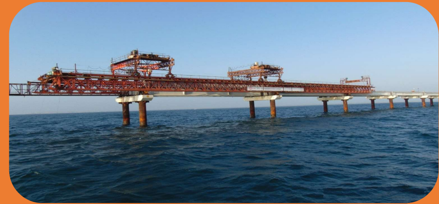
Udangudi Super critical thermal power project in Tamil Nadu
