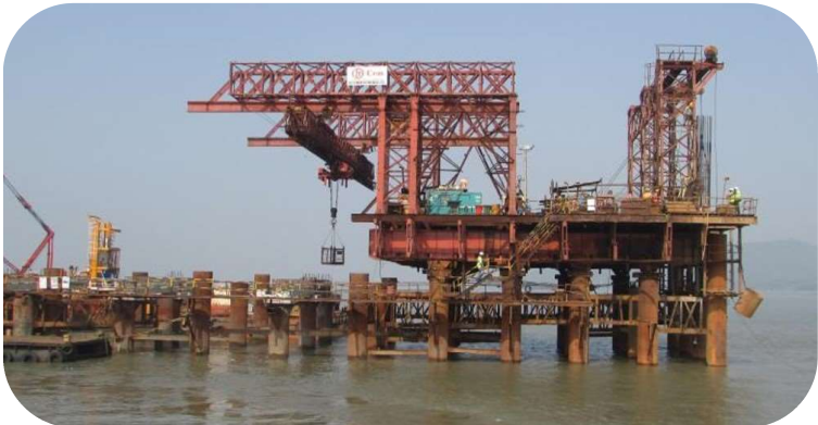
JNPT, Liquid Jetty in Mumbai, Maharashtra
