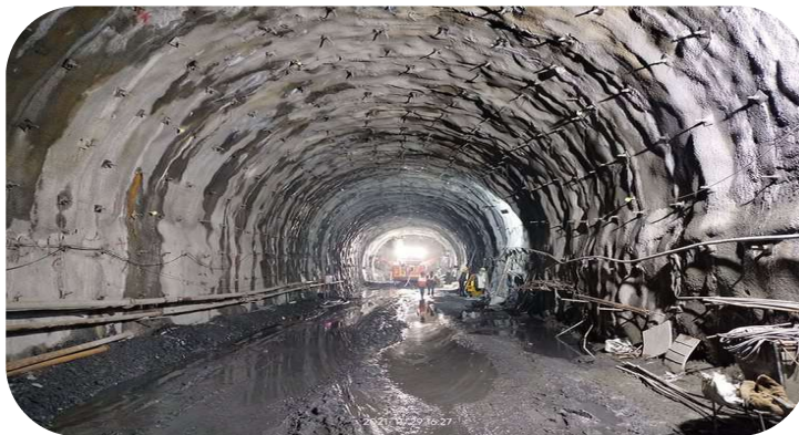
Sivok Rangpo railway tunnel project
