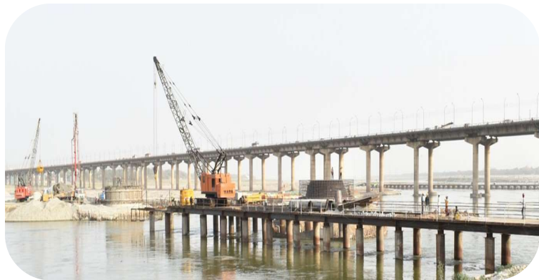
Ganga Steel bridge in Uttar Pradesh
