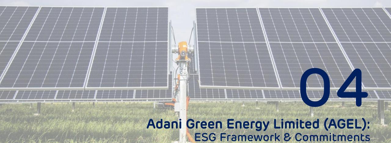
Photo: AGEL's Solar-Wind Hybrid plants at Jaisalmer, Rajasthan (bifacial modules with horizontal single axis trackers)
