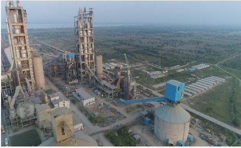
Industrial Plants, Factories & Warehouses
