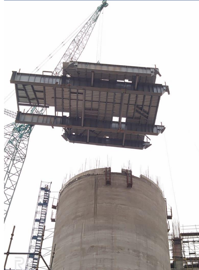
Fly Ash Silo Roof Top Structure erection - Structure pre-assembled at ground and lifted in single piece with 250T crawler crane
