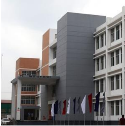
Progress Apparel, Bangladesh
