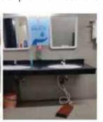
In-house fabricated foot operated sanitizer dispenser, wash basins & motion sensor taps
