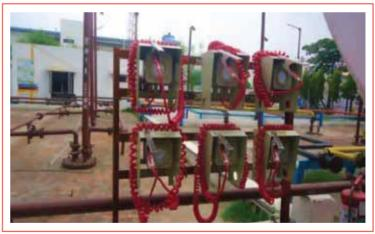
Earth Rite Relay System automation for solvent unloading
