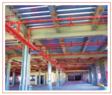
Automatic Foam Sprinkles System installed with QBD & IR3 detection
