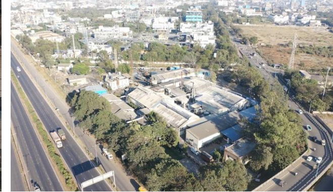
Our Ankleshwar Facility - Gujarat
