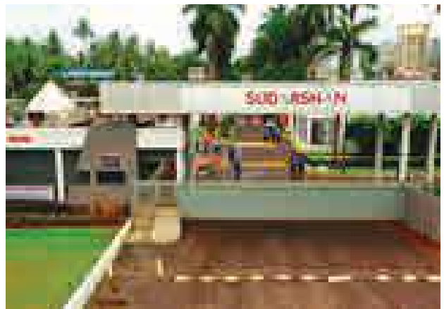
Sudarshan Chemical Industries, Roha Main Gate
