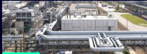
Electrification, Automation & Digitalization solutions
