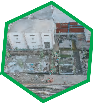
GACL Dahej Caustic Soda Expansion
