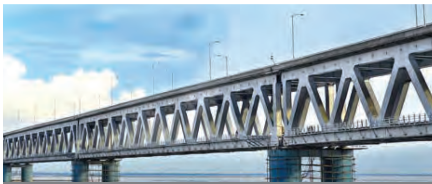
Bogibeel bridge over brahmaputra river in assam coated with AP-PPG Coatings, EPC contractor HCC
