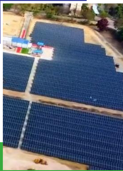
6.5MWp Ground Mounted Project at Raigarh, Chhattisgarh
