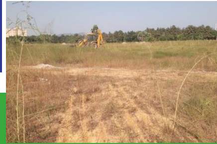
78MWp Ground Mounted Project at Tamnar, Chhattisgarh
