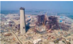
2X660 MW at Rampal, Maitree, Bangladesh-BIFPCL
