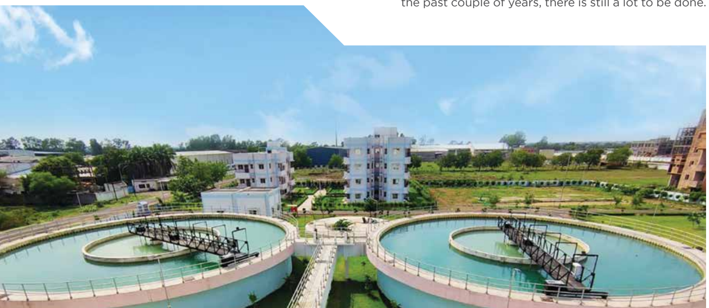
Dewas Industrial Water Supply Project
