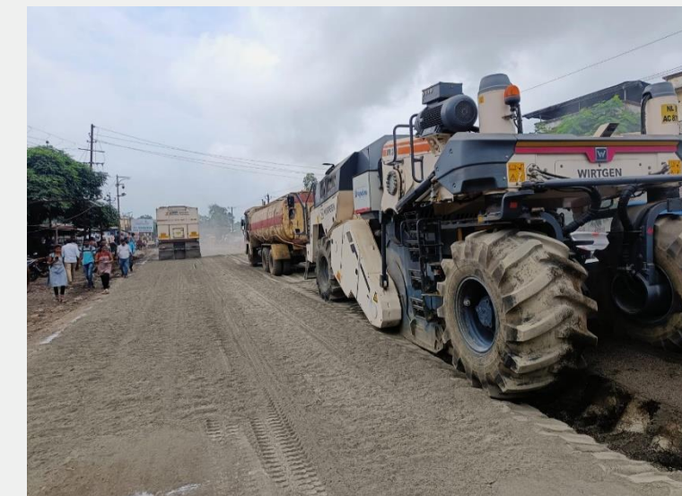
Pulverization of soil with Recycler
