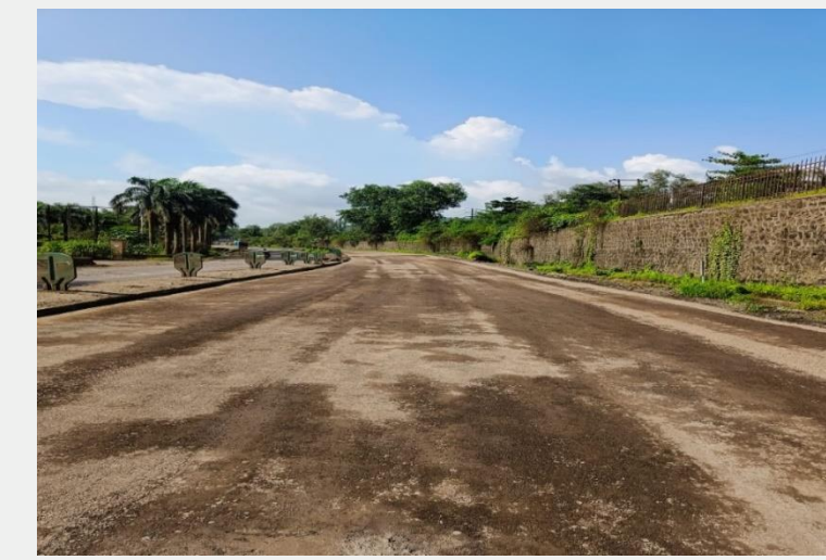
Final surface after Compaction
