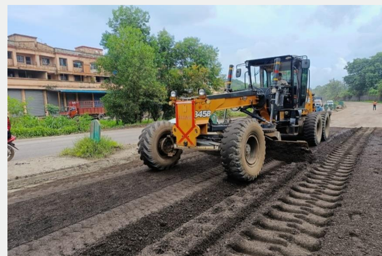
Grading & Profiling with motor Grader
