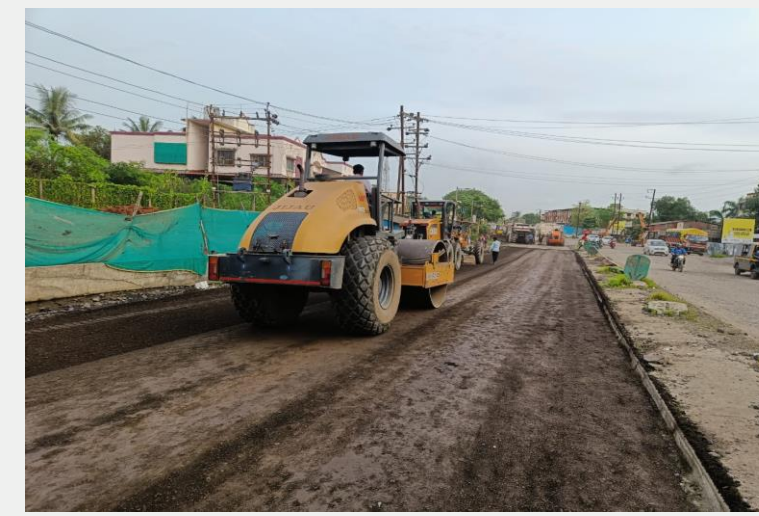
Compaction by Soil Compactor
