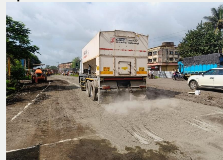
Cement Spreading by Microprocessor Controlled Spreader Truck
