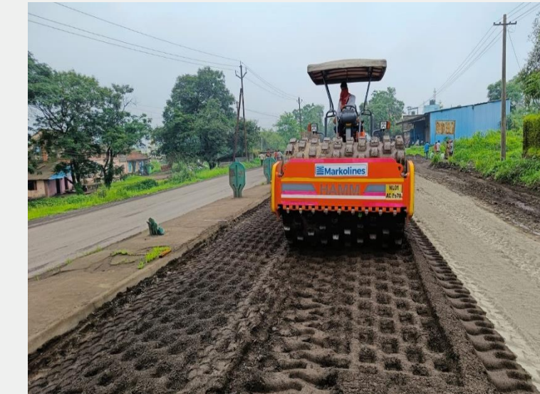
Compaction by Pad Foot Roller
