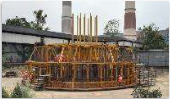
Slipform erection (35 → 25) days
