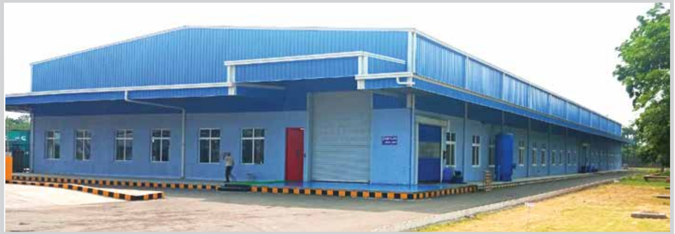
New Plant Addition- Ojas Block
