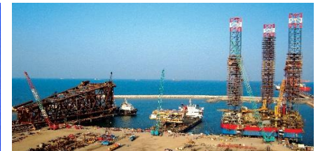
Fabrication Facility, Oman
