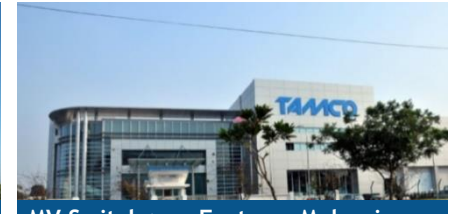
MV Switchgear Factory, Malaysia
