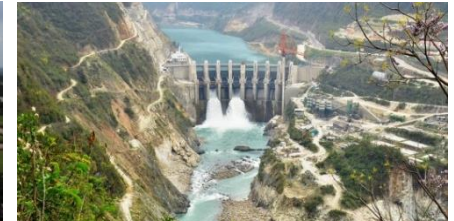
Srinagar Hydro Electric Plant
