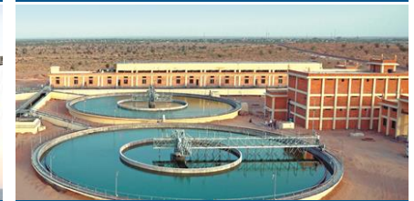
Water Treatment Plant, Barmer
