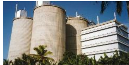
Bulk Cement Terminal, Colombo
