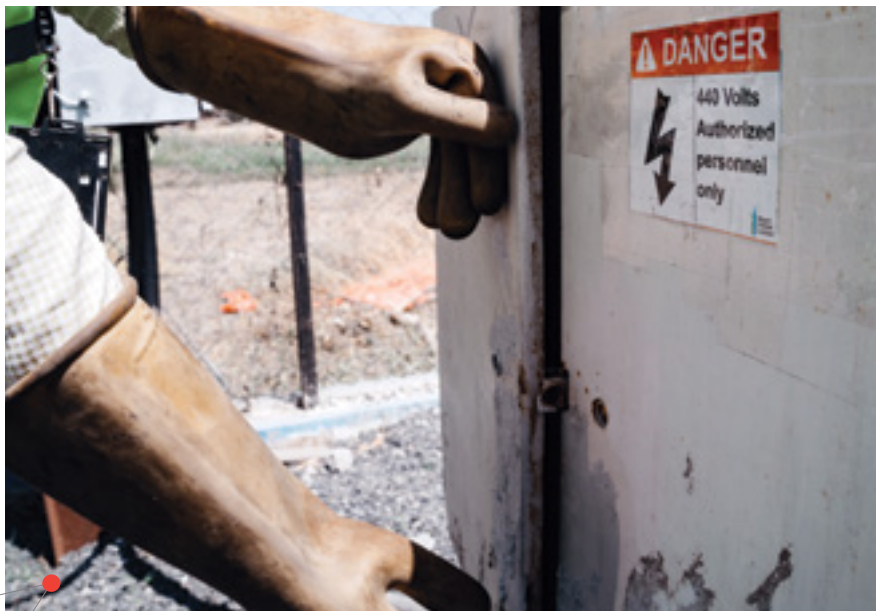
Safe and Secure generator set at tower site
