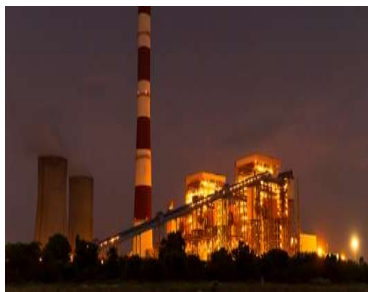
De-NOx, Boiler upgrades; Turbine rotor from STEAG, Tata Power, JSW Steel, Mahagenco
