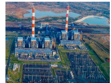
Boiler fly ash erosion execution Unit #2 Adani Tiroda 2x660MW - Chinese OEM
